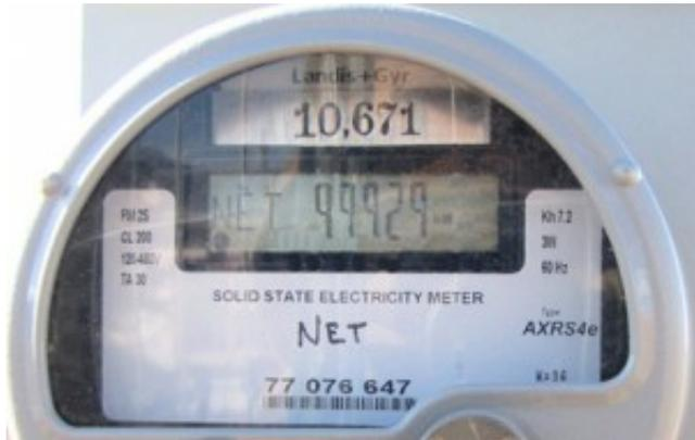
This NET meter started at zero Kwh and now reads 99929, or minus 71 kwh, after a month of recording the electricity coming and going through it.
